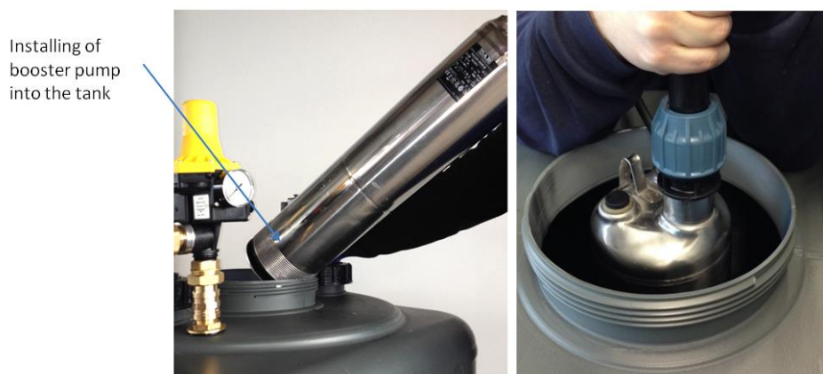
Figure 7: installation of booster pump into tank
